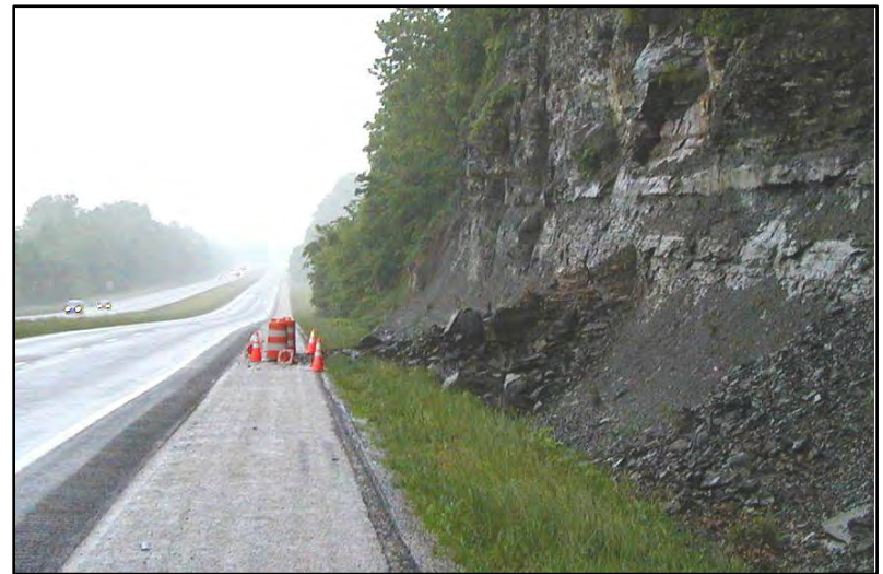
Figure 48 Rock slide along the Bluegrass Parkway. Source: Kentucky Geological Survey.
