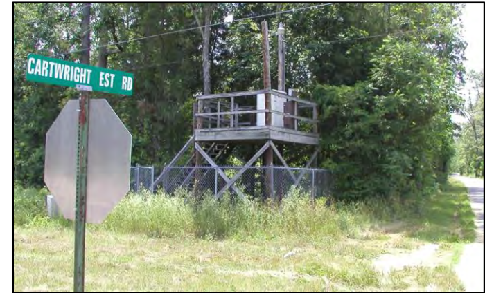
Figure 23 Utilities raised out of Floodplain. Source: LTADD c. 2007.
